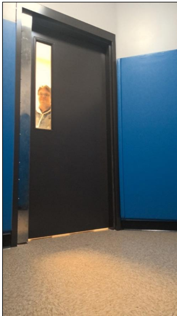
Image 40: Child's view while inside a registered seclusion room, looking out to observation window/closed door where a staff member would observe them from outside the locked room. An adult man approximately 5 feet 9 inches tall stands where a staff member would observe the child. The observation window – a narrow rectangle approximately 6 inches wide and 24 inches long – is a common design for seclusion rooms in Minnesota. SWWC Education Learning Center – Montevideo, MN
