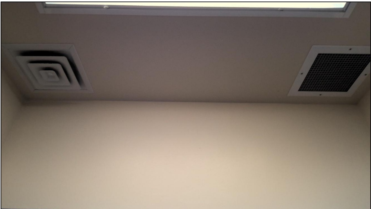
Image 45: Seclusion room ceiling ventilation system, in compliance with Minnesotan statute. Bemidji High School – Bemidji, MN
