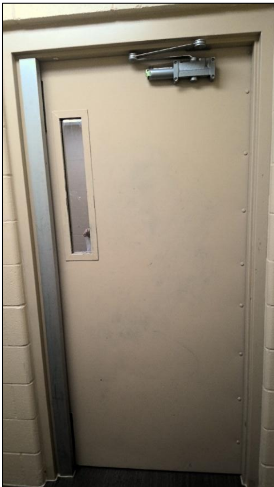
Image 39: Child's view while inside a registered seclusion room, looking out to observation window/closed door where a staff member would observe them from outside the locked room. The observation window – a narrow rectangle approximately 4 inches wide and 24 inches long – is a common design for seclusion rooms in Minnesota. The long silver strip on the left side of the door is the magnetic (keyless) locking mechanism. Alliance Education Center – Rosemount, MN
