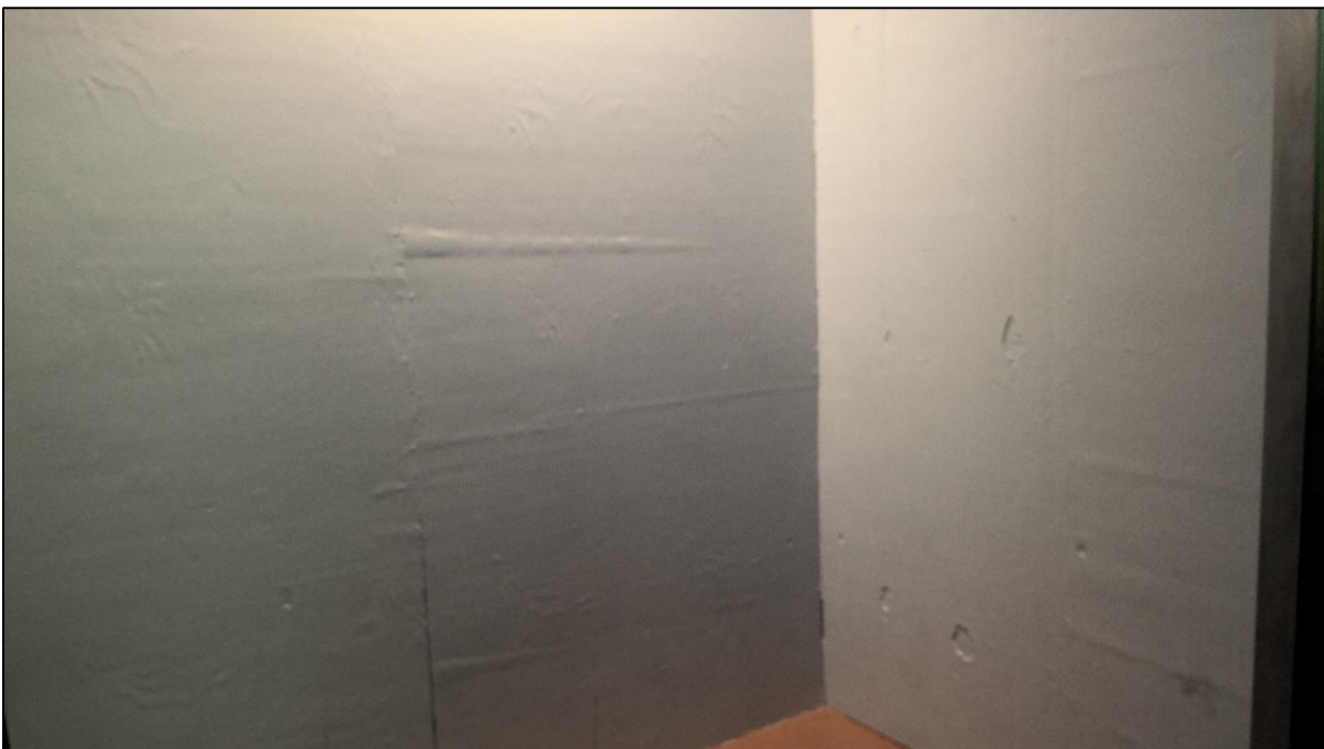
Image 35: Seclusion room walls with small holes/indents, indicating the walls are not tamperproof. Franklin Elementary School – Rochester, MN
