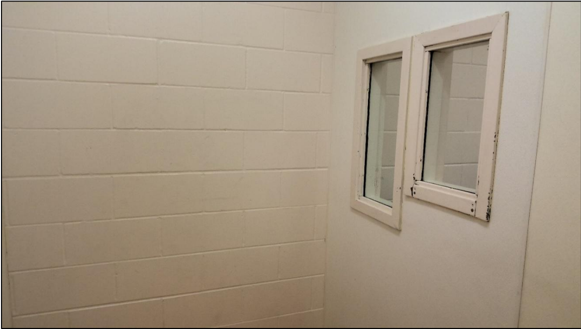
Image 3: Registered seclusion room with cinder block walls and metal window frames with chipped paint in Isanti Intermediate School - Isanti, MN
