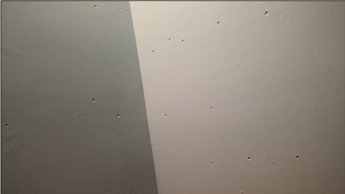
Image 34: Registered seclusion room walls with small holes/indents, indicating the walls and fixtures are not tamperproof or clean as required by Minnesota statute. Franklin Elementary School – Rochester, MN.
