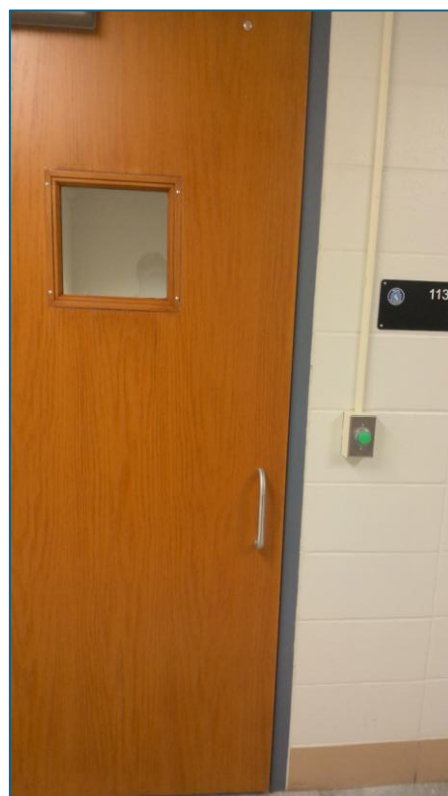
Image 46: Locking push-button mechanism outside of the seclusion room. Webster K-12 – North St. Paul, MN
