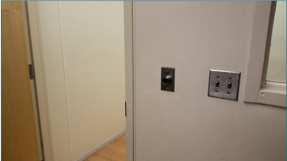
Image 52: Locking push button mechanism outside of seclusion room door. Isanti Intermediate School – Isanti, MN
