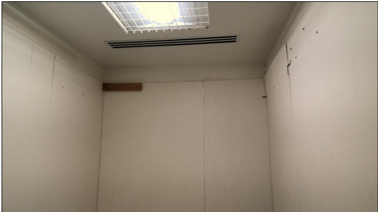
Image 33: Detail of seclusion room ceiling with grated light fixture and unsecured wall panels that have cracks and gaps between the panels. Additional screws and wood bracing runs along the top of the wall panels. Cambridge Intermediate School – Cambridge, MN
