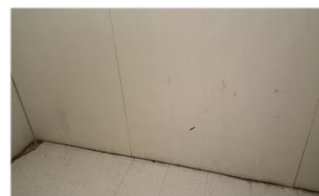
Detail of seclusion room floor with damaged and unclean floor and walls, mold or water damage appearing in cracks between floor and walls. Cambridge Intermediate School – Cambridge, MN
