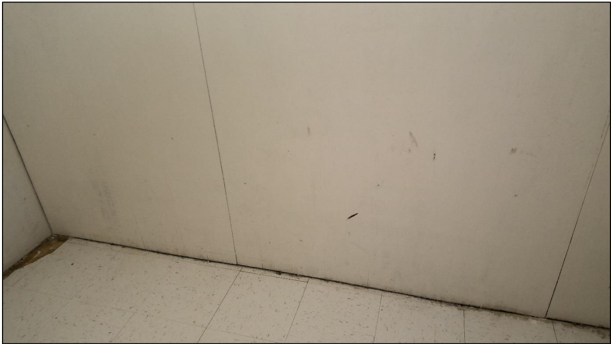
Image 32: Detail of seclusion room floor with damaged and unclean floor and walls, mold or water damage appearing in cracks between floor and walls. A piece of the floor tile is missing, leaving a jagged gap in the floor surface. Cambridge Intermediate School – Cambridge, MN
