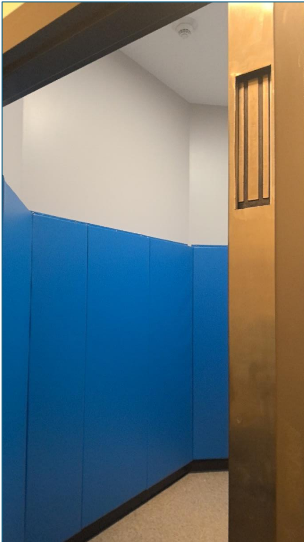
Image 48: Image Magnetic door lock running along the right side of the seclusion door. SWWC ELC - Montevideo, MN
