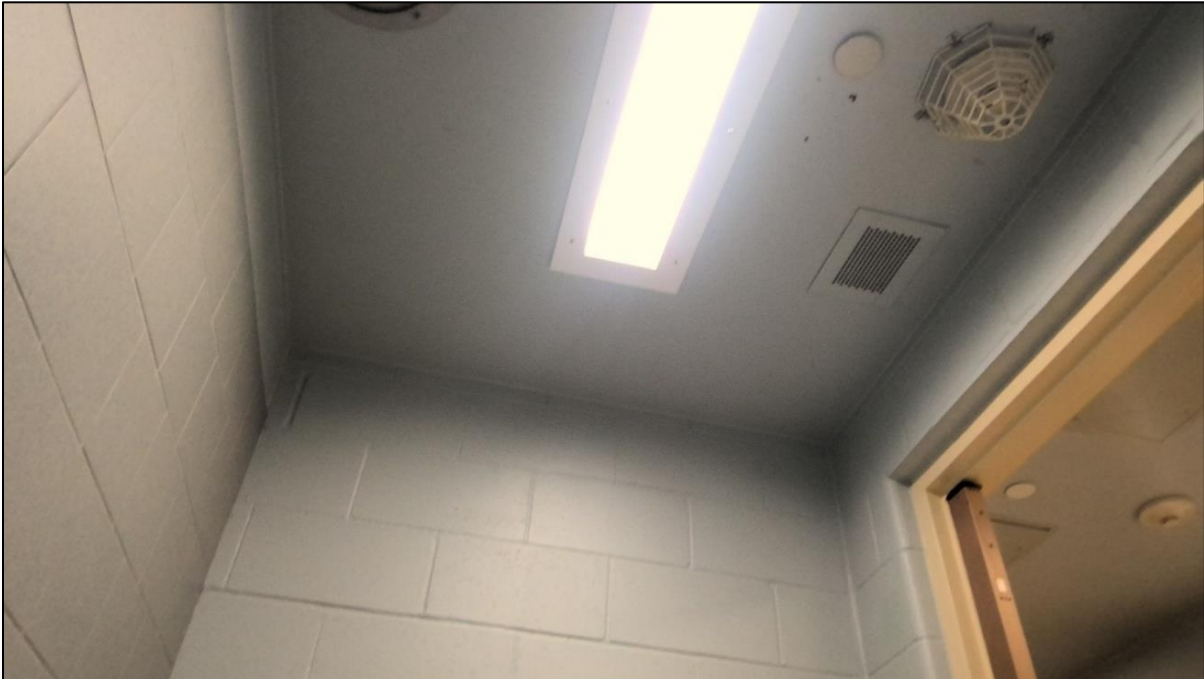
Image 44: Seclusion room ceiling with secure ceiling, tamperproof light, and smoke alarm with a grate around it on ceiling. River Trail Learning Center – Coon Rapids, MN
